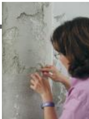
As well as its decorative function, plaster protects masonry against humidity.
